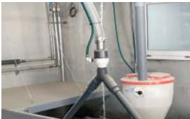
Distribution valve with the AWI® injector (Automatic Water Injection).
